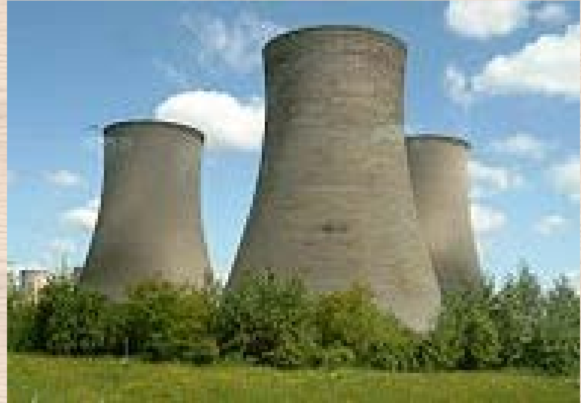
Hyperbolic shaped cooling tower
